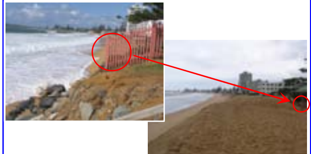
Collaroy/Narrabeen Beach before (left) and after (right) replenishment. View from Wet herill St looking South.
